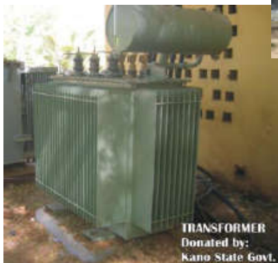
A 33KVA Transformer Servicing the Hospital
